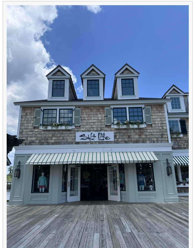
Exterior of the new SALT LIFE retail store in North Myrtle Beach, South Carolina.
