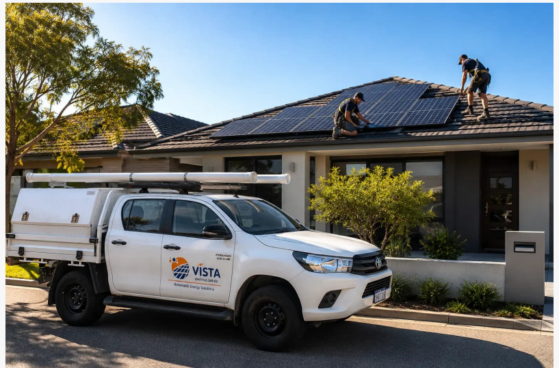
Top Perth Solar Installer
