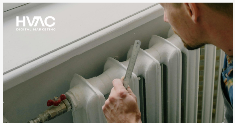
HVAC Employee adjusting hose
