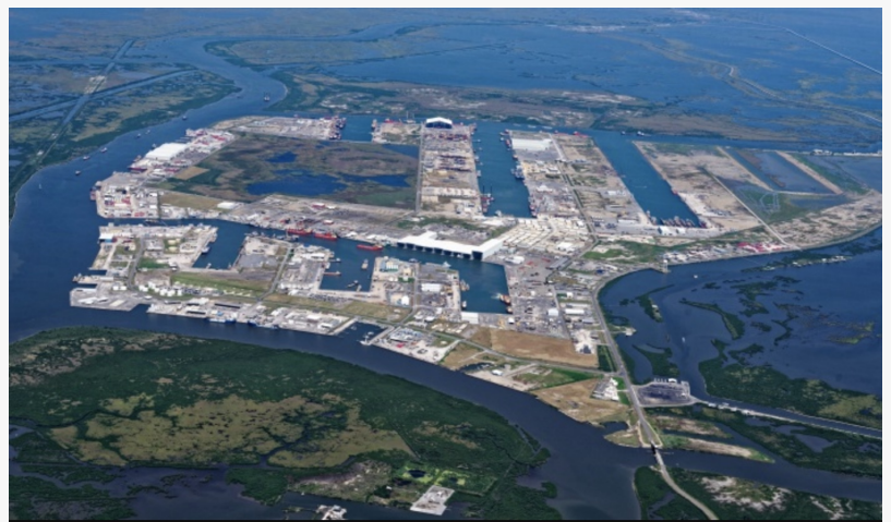
Port Fourchon is a multi-use coastal port that functions primarily as a land base for multiple offshore energy support service companies.
