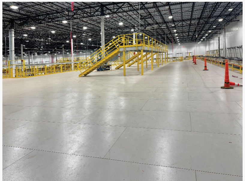
ResinDek flooring panels on multiple platforms with varying elevations
