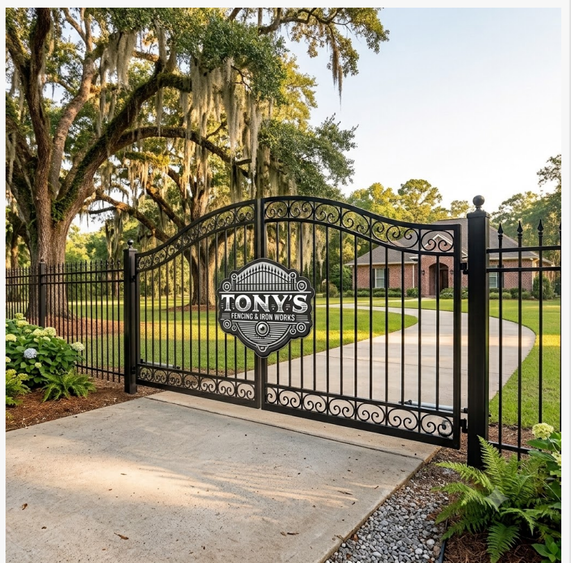
Custom ornamental iron gate installation by Tony's Fencing & Iron Works for secure, stylish residential access in Southeast Louisiana.
