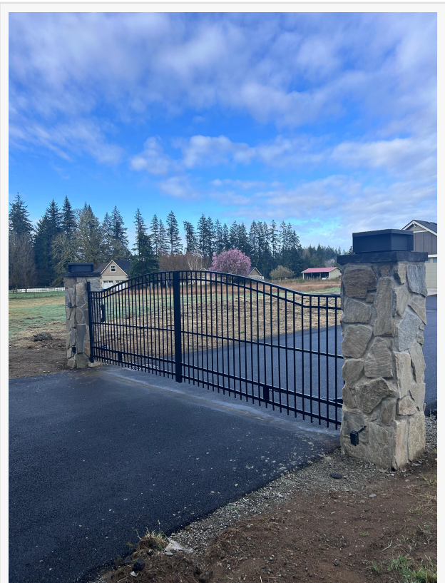
Custom electric driveway gate installed by Interactive Gates & Security in the greater Seattle area — serving Gig Harbor, Bellevue, Woodinville, Issaquah, and all of King, Pierce, and Snohomish Counties.
