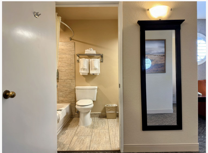
Updated guest bathroom completed at the Best Western Escondido Hotel. Level 3 Construction was responsible for the renovation work.
