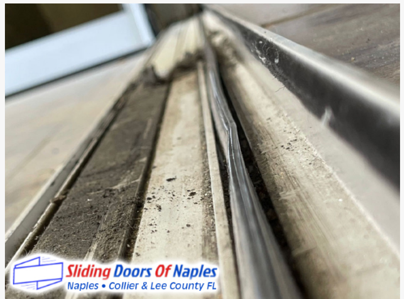
Sliding Door Track Repair
