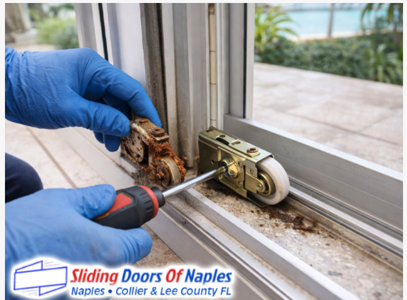
Sliding Door Rollers Replacement
