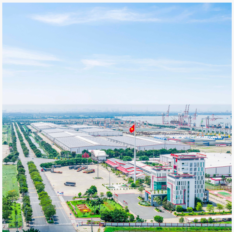
Smart Green Port initiatives implemented across Long An International Port
