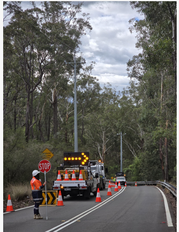
Black Label Traffic supporting civil road works with professional traffic control at an active Sydney work zone.
