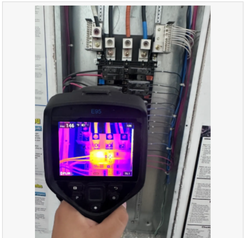
Electrical Thermography Level III
