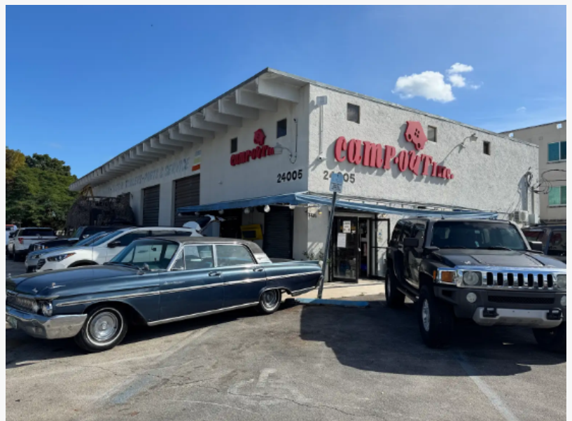
Commercial Building Inspection
