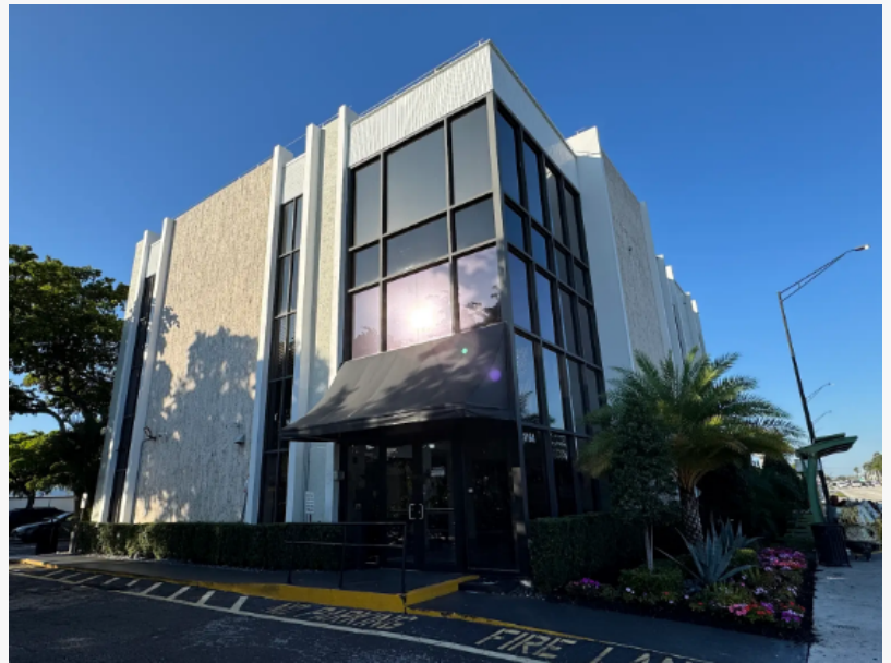
Building Recertification Inspections
