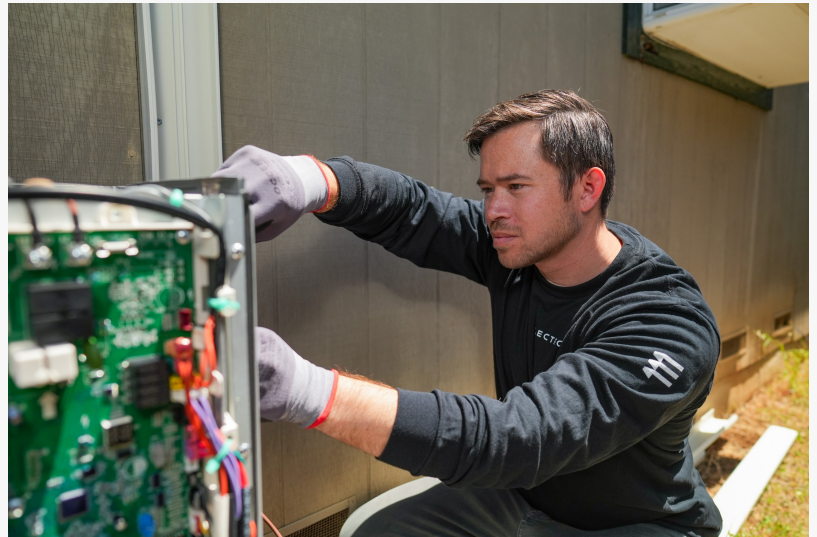
Contractor installing a heat pump outside a house
