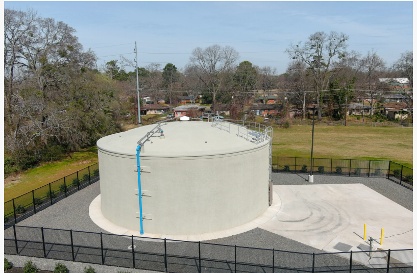
The Preload team began work on the Shreveport tank in late November 2024, wrapping up in March 2025.
