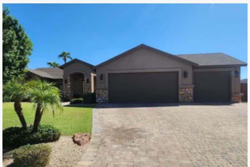
Garage Door Installation
