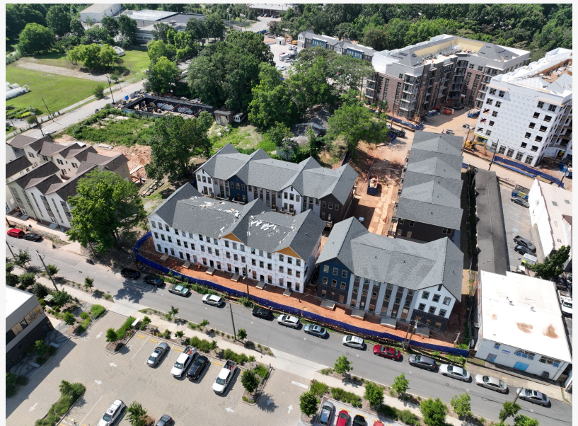
Woodrow House advances along Atlanta Beltline's Westside Trail
