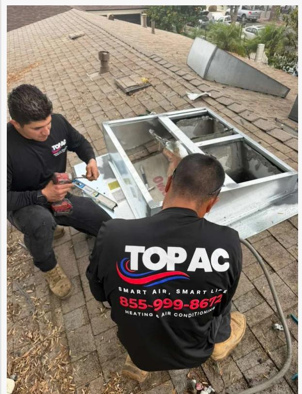
TOP AC Inc. certified technicians completing an HVAC installation in Los Angeles. Same-day service available across 30+ LA neighborhoods. CSLB #959168.
