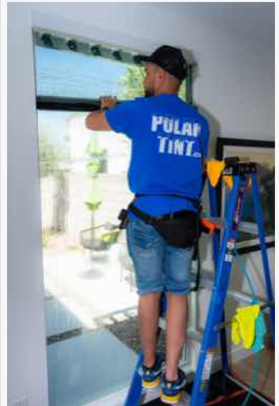
A Polar Tint Summerlin technician installing residential solar window film.
