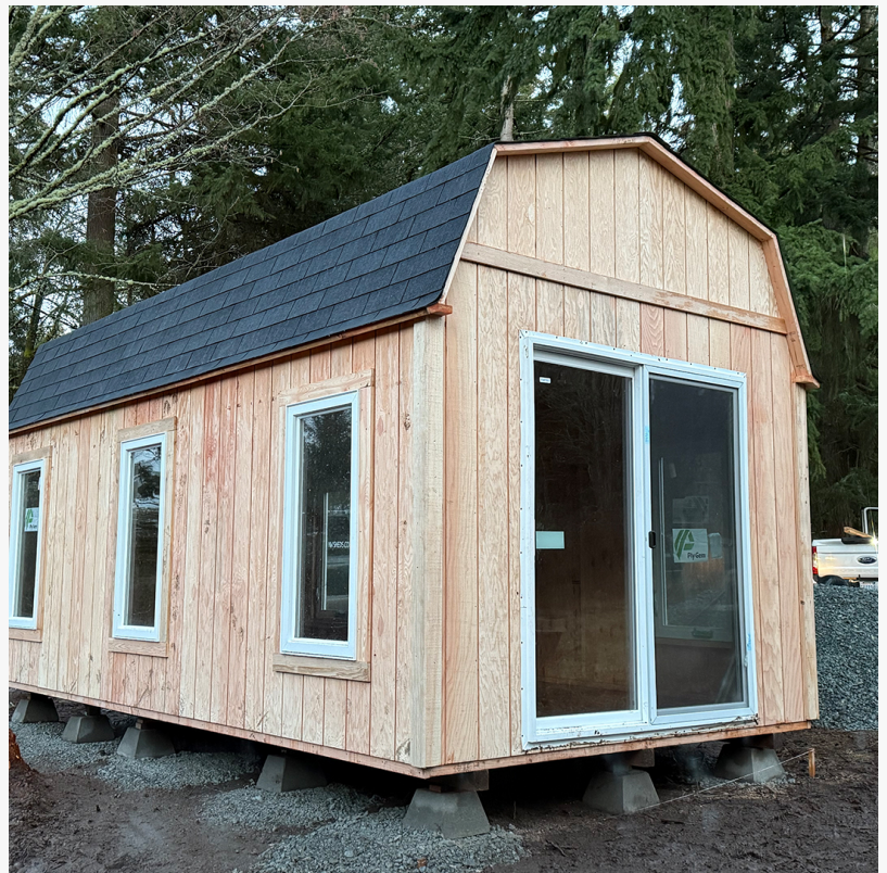
shed installation WA,
