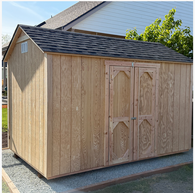
custom shed installation Seattle WA,
