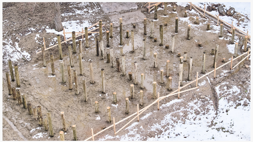
Ne's foundation: 105 timber piles, built without concrete. Photo: Hiroki Kawata
