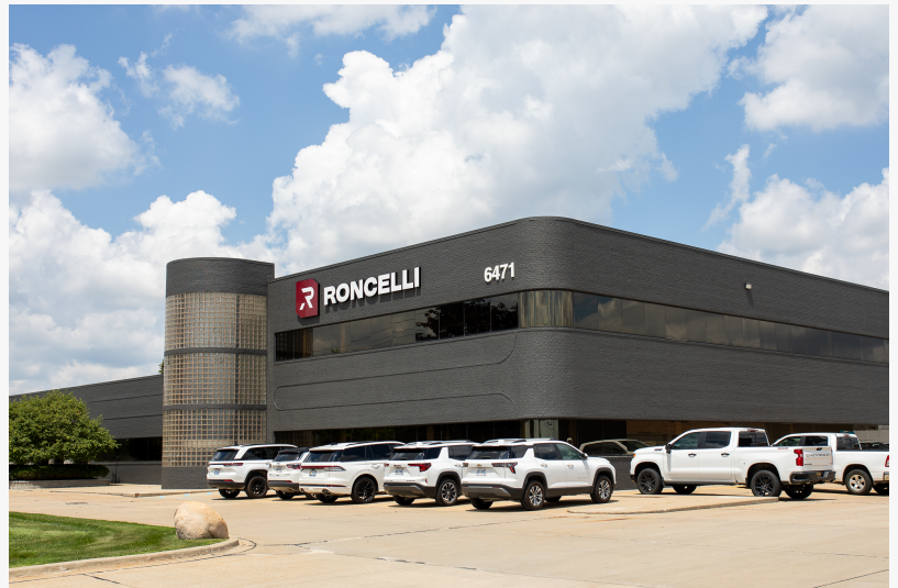
New Roncelli Headquarters in Sterling Heights
