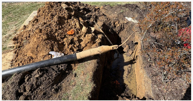
Underground water line repair with exposed pipe in construction trench
