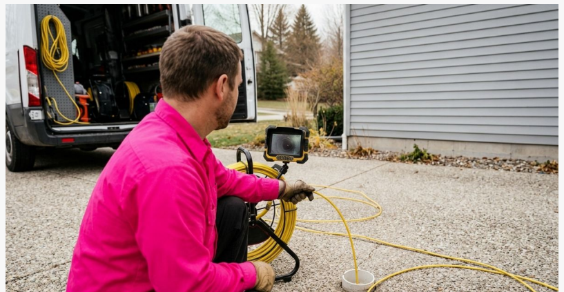
Underground sewer camera inspection service for detecting pipe issues
