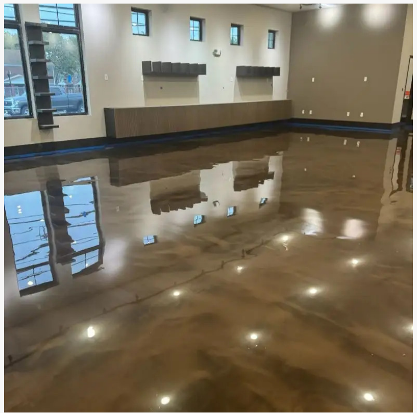
Grind and Seal Epoxy Flooring
