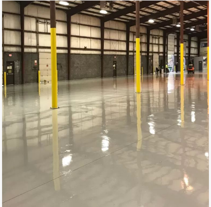
Warehouse and Distribution Center Flooring
