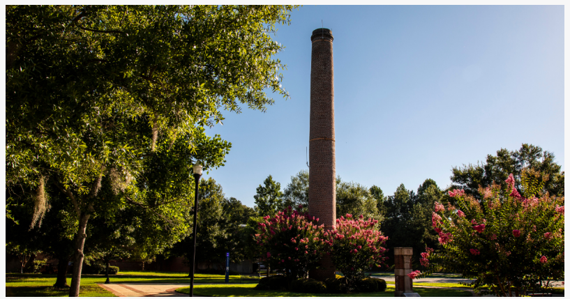
Albany State Chimney
