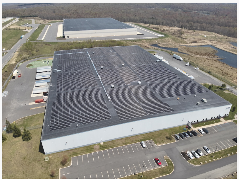
2.8 MWdc rooftop solar project in Covington Township, PA.
