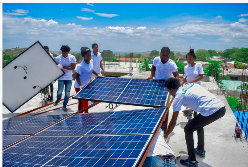
Solar Apprentices installing solar energy at school
