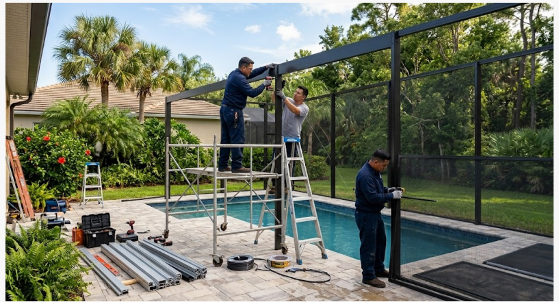
Pool Screen Enclosure in Altamonte Springs, FL
