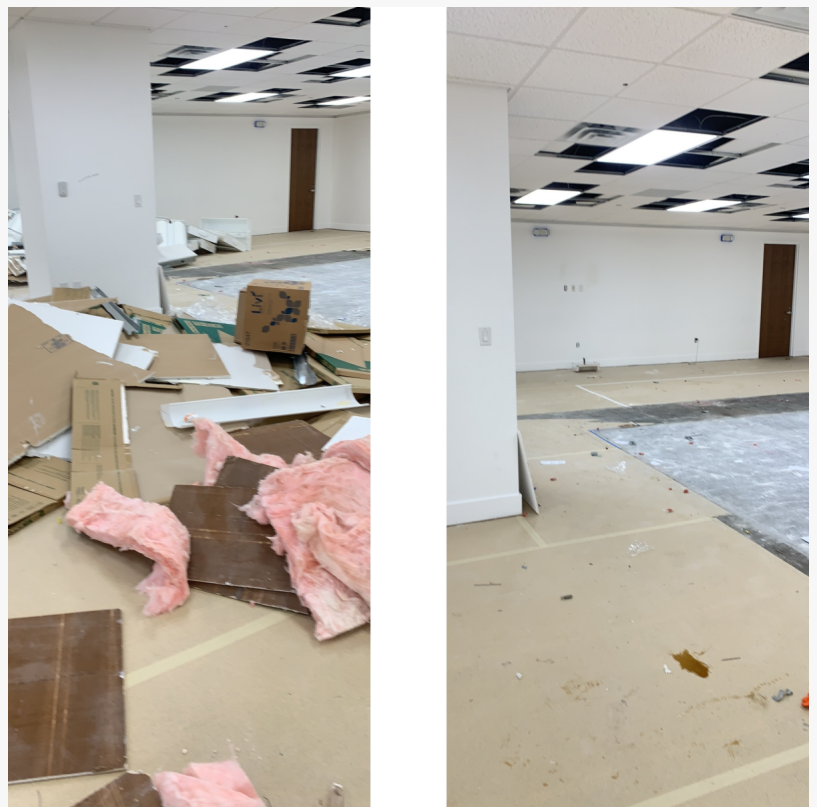
Before and after commercial property cleanout completed by XS Trash.
