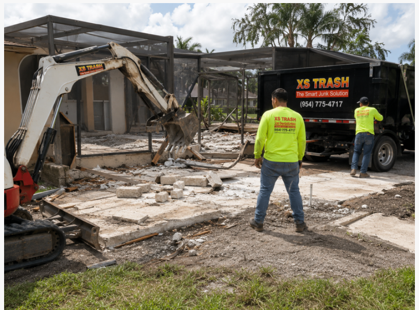
XS Trash removing heavy debris using bobcat equipment during a commercial property cleanout.
