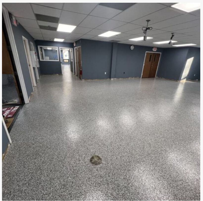
Warehouse Epoxy Flooring System
