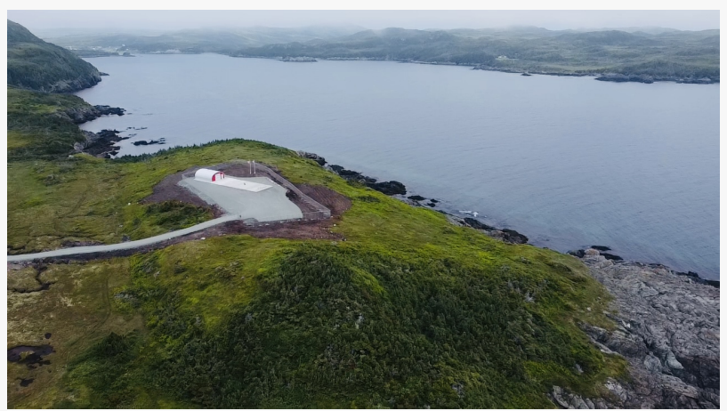
NordSpace's Atlantic Spaceport Complex (ASX) SLC-02 Under Construction
