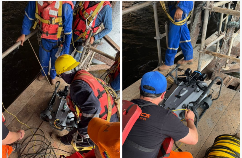
INMARVENCO technicians prepare the CHASING X industrial ROV for an underwater pile inspection in Venezuela's Caroní River.
