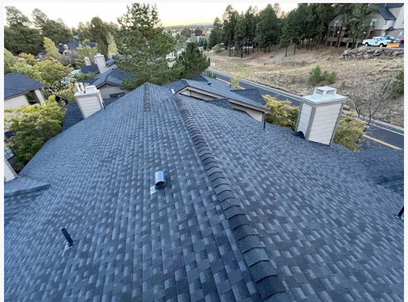
ProWest Roofing, Arizona
