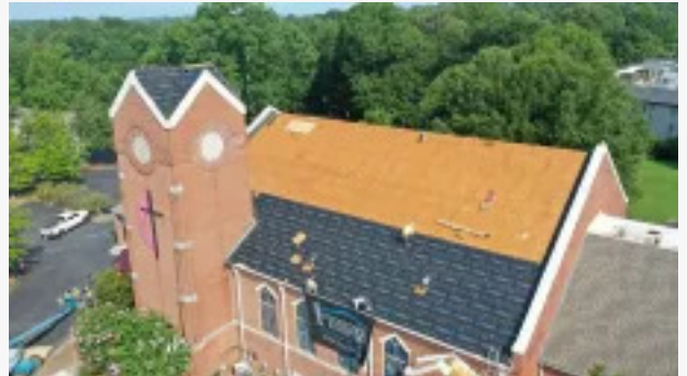
Commercial Roofing Services
