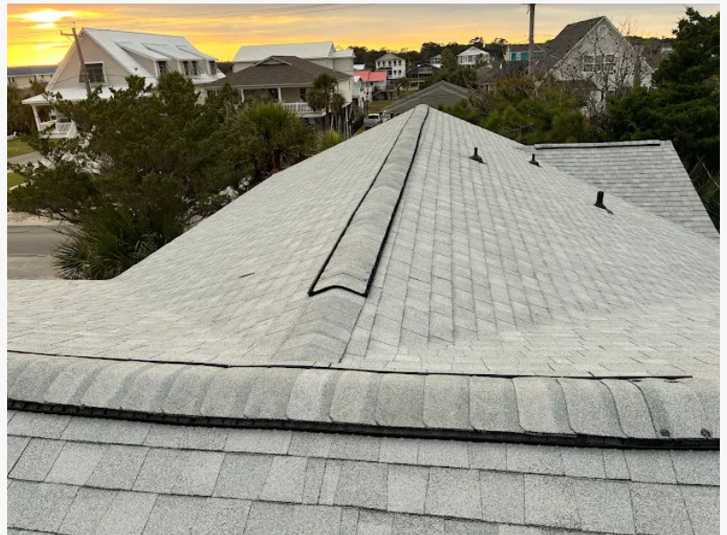
Roof and Damage Restoration Company
