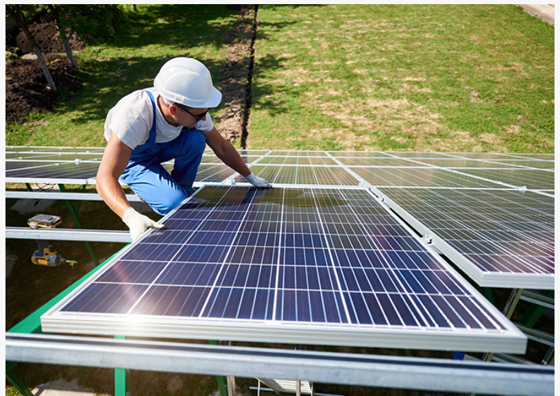
Businesses Solar Installation in Pitkin
