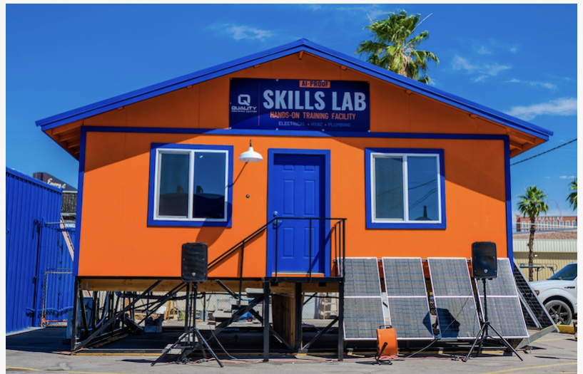
QTC builds its curriculum around real job-site conditions, including hands-on experience in a residential skills lab built as an actual house.
