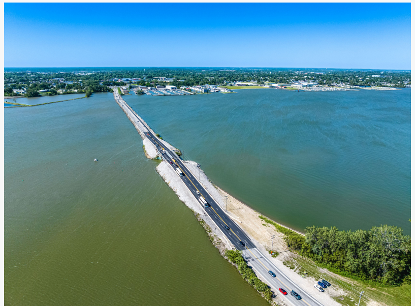
Acrow Bridge at Cedar Point Ohio
