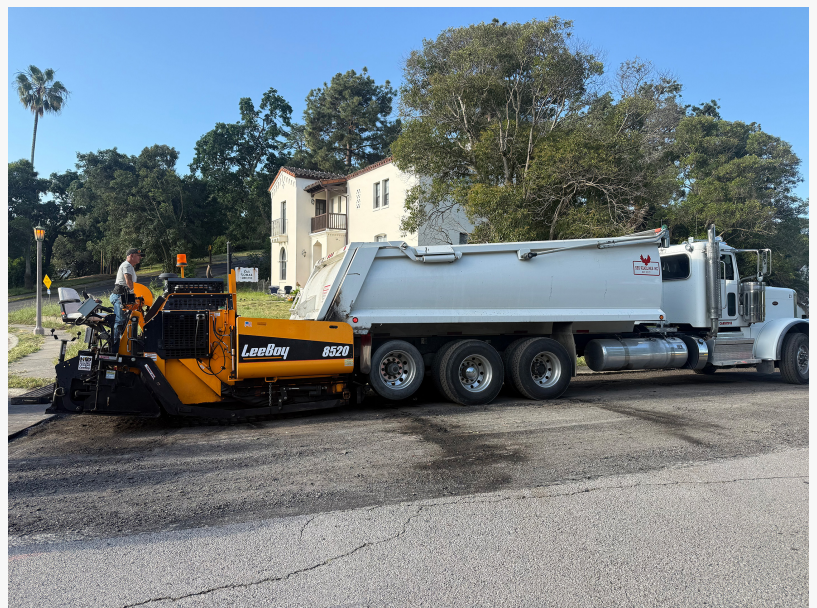
A 2025 LeeBoy 8520 commercial asphalt paver receives hot mix from an SBS Roadlines Inc. delivery truck during a North Bay Grading and Paving roadway resurfacing project in Novato, California. The LeeBoy 8520 anchors the Santa Rosa paving contractor’s comm
