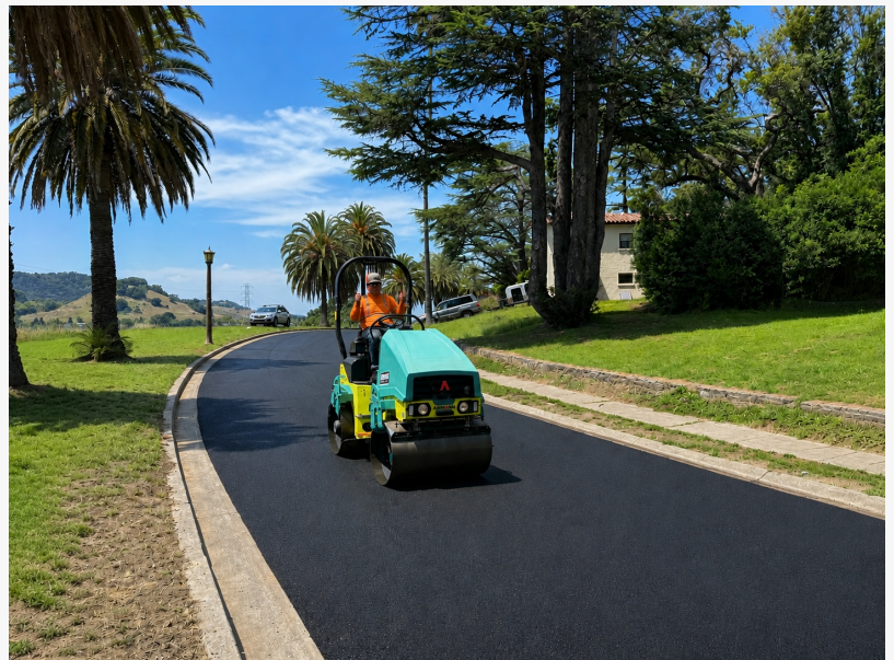
A North Bay Grading and Paving crew member operates a double-drum vibratory asphalt roller during a private roadway resurfacing project in the Sonoma County area.
