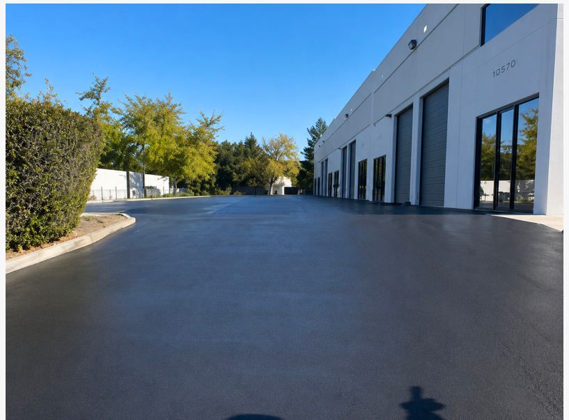
A completed section of newly paved roadway at Hamilton Field in Novato showcases the finished work of North Bay Grading and Paving, including a fresh double-yellow centerline, white speed bump striping and a smooth compacted asphalt surface. The Santa Ros
