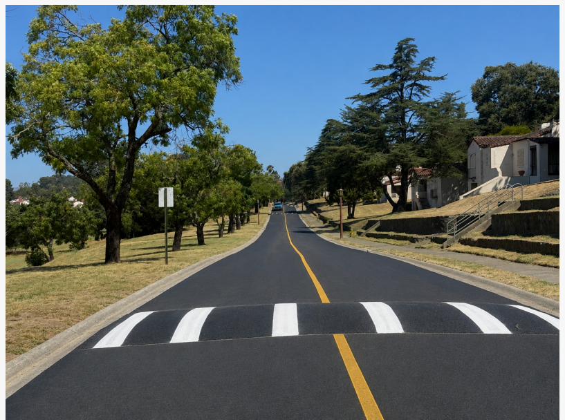
A newly resurfaced apartment complex parking lot completed by North Bay Grading and Paving in the Sonoma County area. The Santa Rosa paving contractor regularly delivers multifamily property paving, HOA parking lot resurfacing, roadway resurfacing and asp
