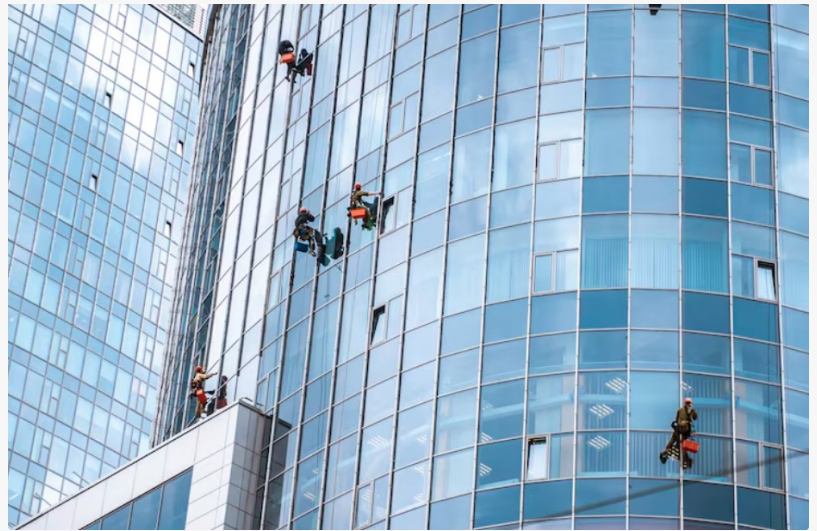
Emergency Glass Repair,
