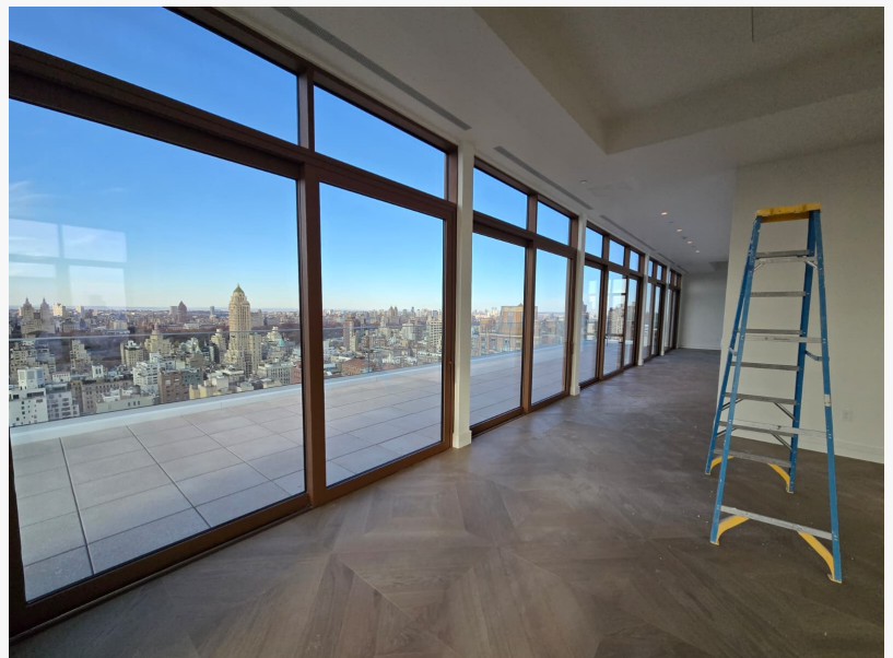
Glass Repair in NY,
