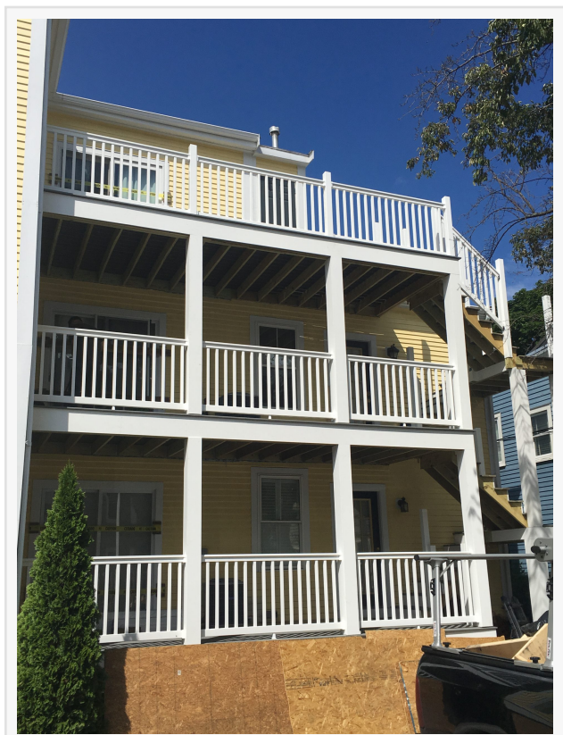
Brookline whole home renovation contractor
