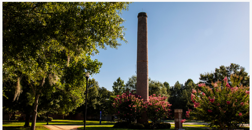
Albany State Chimney
