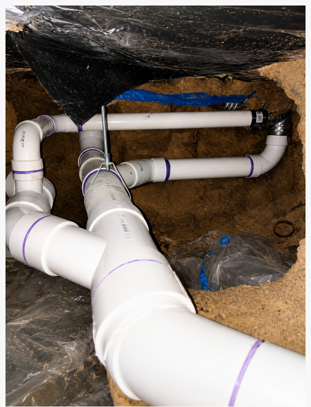
New PVC drain piping installed in a commercial crawl space as part of a professional sewer line repair and drain system upgrade by Plumbing System Pros.
