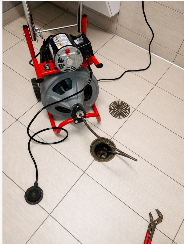
A professional drain cleaning machine is used to clear a clogged floor drain, restoring proper drainage in a commercial restroom.
