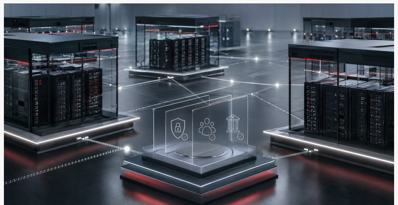
Federated Sovereign Node infrastructure supports sovereign AI and cloud control across qualified institutions.
