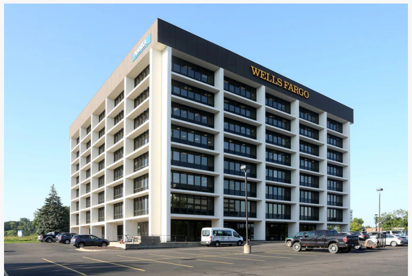
MetroPointe Office Campus
