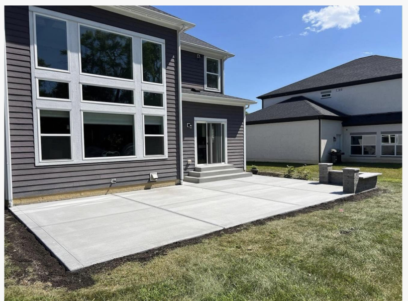
New Concrete Patio with Seating Wall
