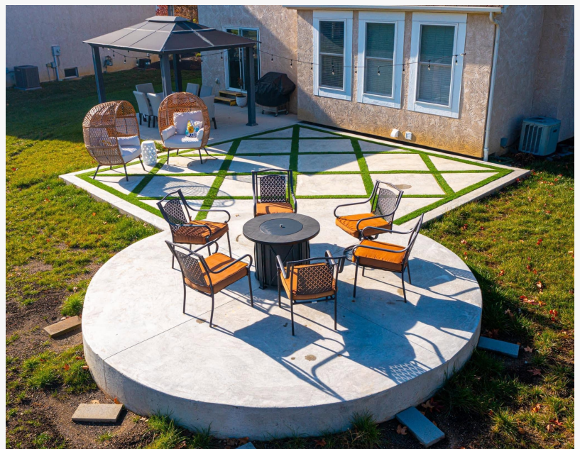
New Concrete Patio
