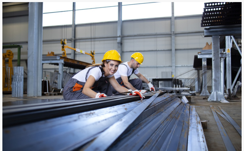
contract metal fabrication
