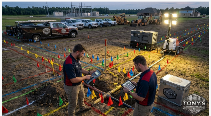
Fence professionals review color-coded underground utility markings before posts and gate supports are installed on a Louisiana property.
