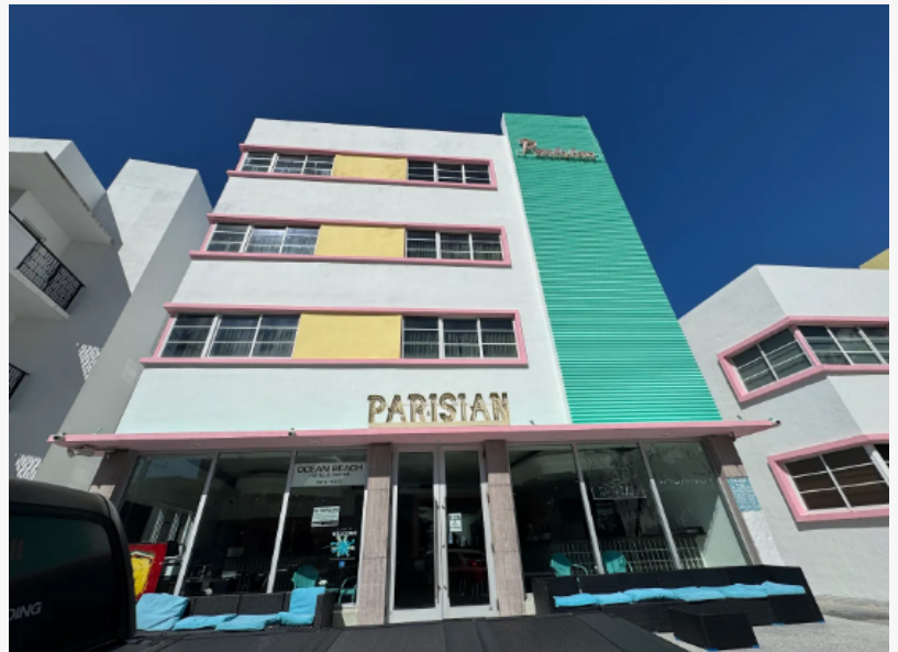
Building Recertification Inspections_
