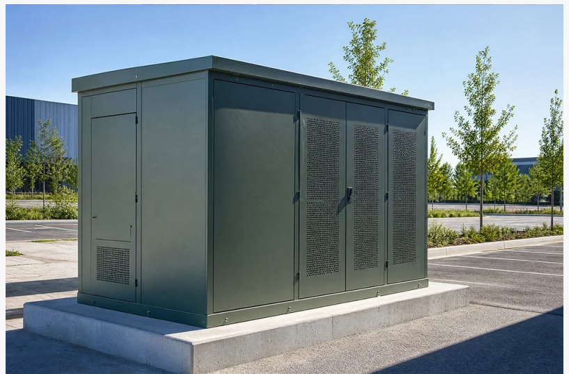
EV Charging Infrastructure
