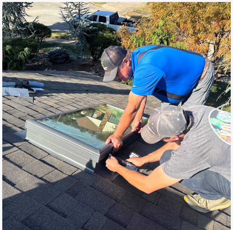
Whirlwind Roofing installing a skylight on an IBHS FORTIFIED roof replacement
